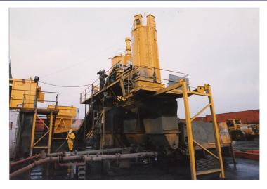
Work involved bulk infilling, grouting and underground work to stabilise redundant limestone mine workings, in two areas of approximately 15 ha. of residential, open space, roads and canals. The scheme was funded by English Partnerships Land Stabilisation Programme
