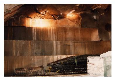
Access to the barrier works in Little Tess and Hurst Cavern were via the existing operational canal system requiring agreement of timetables, methods, emergency procedures and safety systems with Dudley Canal Trust, who continued to use the canal system for tourist trips. Generally barriers were constructed using in-situ reinforced concrete with sacrificial blockwork back shuttering. Concrete was pumped from surface through purpose drilled and cased holes at barrier positions.
